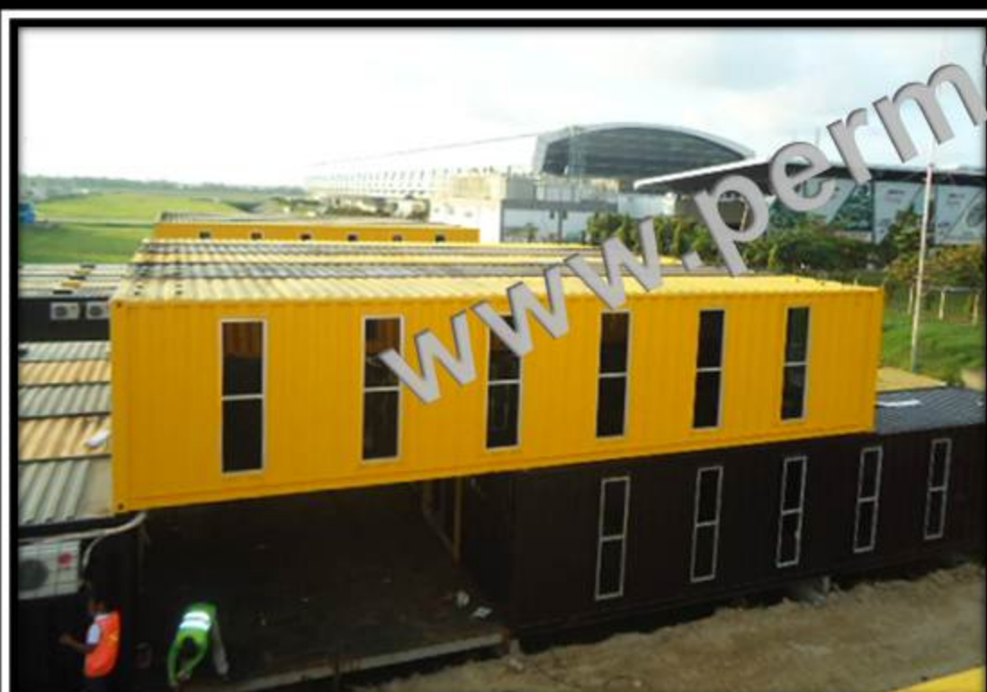
Project Office dan Camp container di Bandara Soekarno Hatta terminal 3
